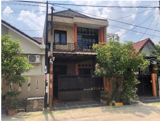
Figure 3. Structure Construction Source: (Khalis, 2022)
