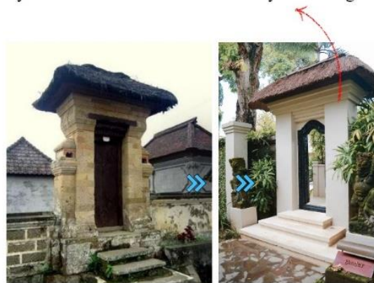
Figure 6. Transforming the makekerep structure into a modern look at Kayu Manis Villa Sanur (Source: analysis, 2021)
