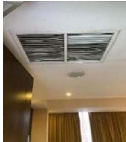
**Gambar 10.** Unit AC Indoor FCU (Kiri) dan Diffuser Return (Kanan)
