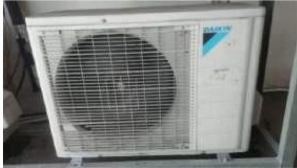
**Gambar 9.** Salah Satu Unit AC Outdoor (CU) Kapasitas 1,5 PK
