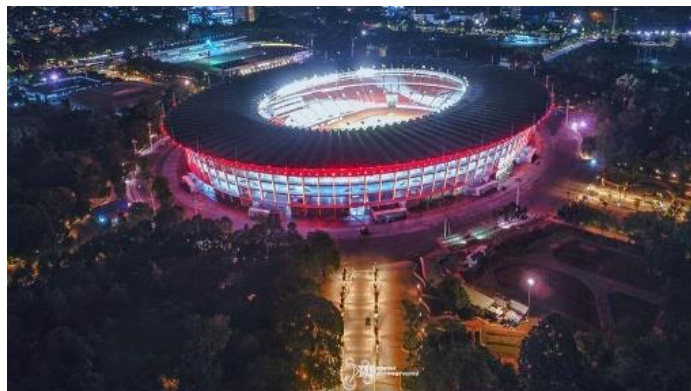
Gambar 1. Tampak Stadion Gelora Bung Karno, Senayan Jakarta Sumber: Data Literatur,2019
