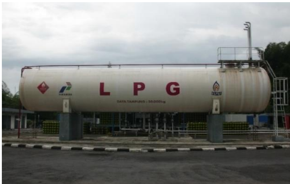
Figure 4. Photographic view of the LPG tank studied in PT Kayu Lima Utama gas station.
