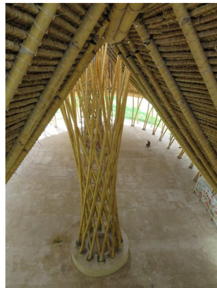
Figure 6. Interior of Three Mountain Building (Widyowijatnoko, 2016)
