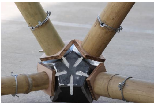
Figure 9. Knock-down connection
