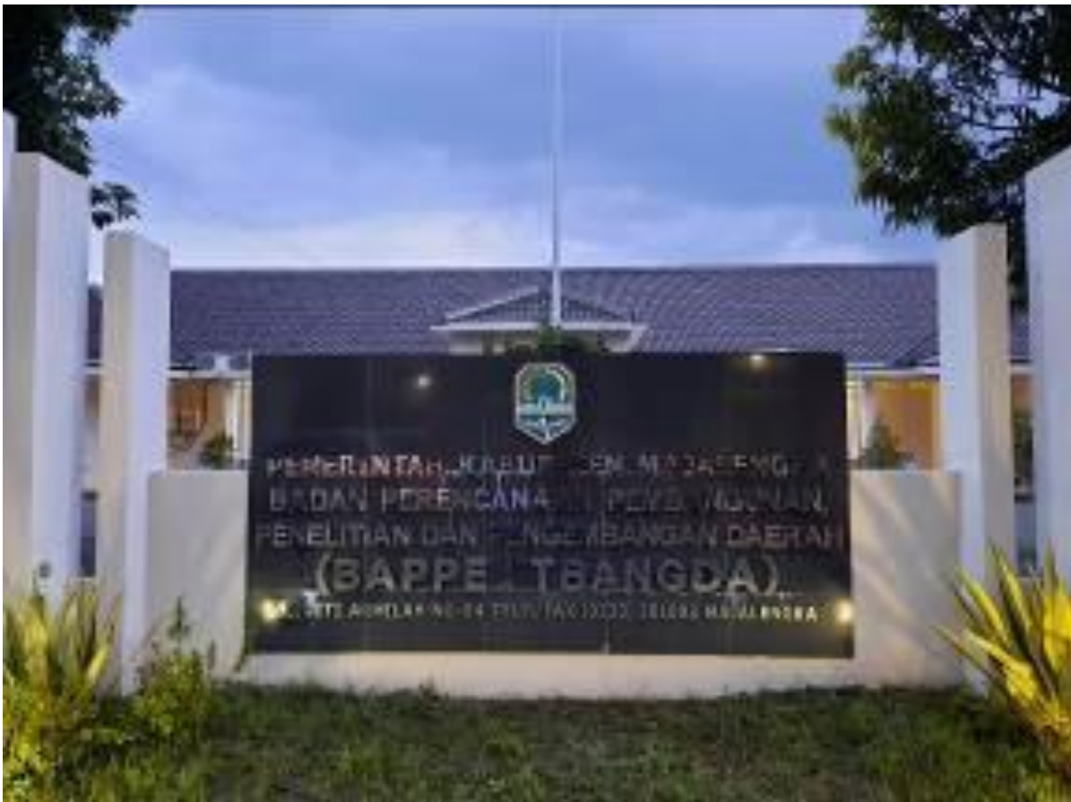
Figure 1. Bappedalitbang office Majalengka Regency Source: Bappedalitbang Kab. Majalengka
