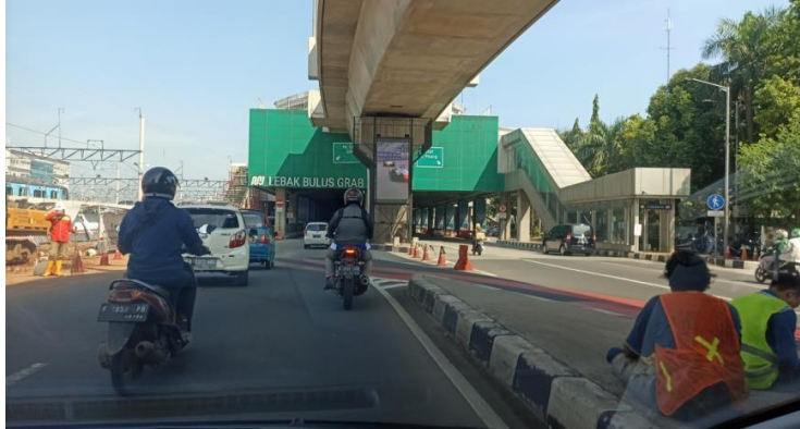
Figures 4. MRT Station Entrance
