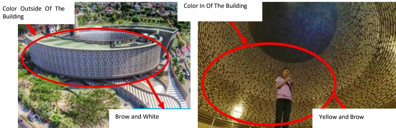
Picture 16. Afied 1 And Ashadi 2 , Use of Interior and Exterior Colors of the Aceh Tsunami Museum, 2021.
