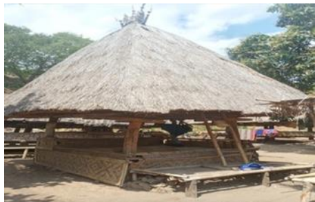
Pic 6. Four-storey traditional house
