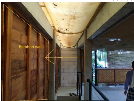
Figure 5 : Wall elements in the house : Bamboo pressed panels Source : Writer, 2023
