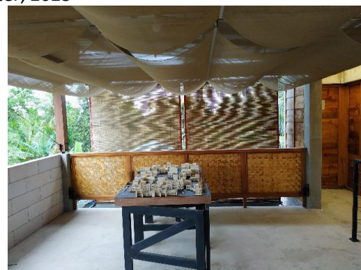
Figure 7 : Roof elements on the house : Fabric ceiling Source : Writer, 2023
