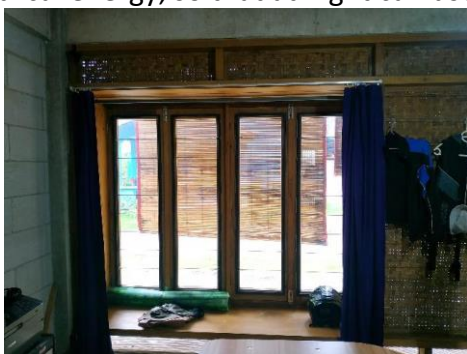
Figure 3 : Opening elements in the house : Glass windows Source : Writer, 2023
