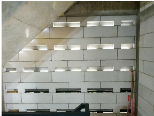
Figure 5 : Wall elements in the house : Hollow bricks Source : Writer, 2023
