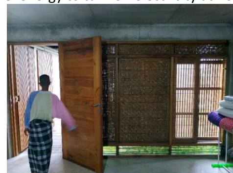
Figure 4 : Opening elements in the house : Wooden door and bamboo window Source : Writer, 2023
