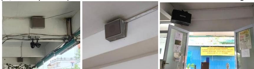
Figure 24. Installation of Speakers in Nursing Homes Source: Author, 2022
