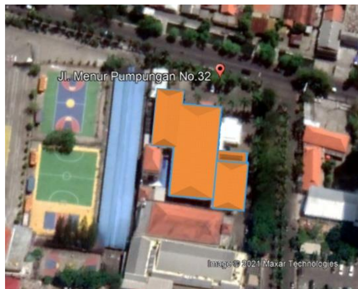
Figure 1. Location of the Regional Library of East Java Province, 2021, Photo from above.
