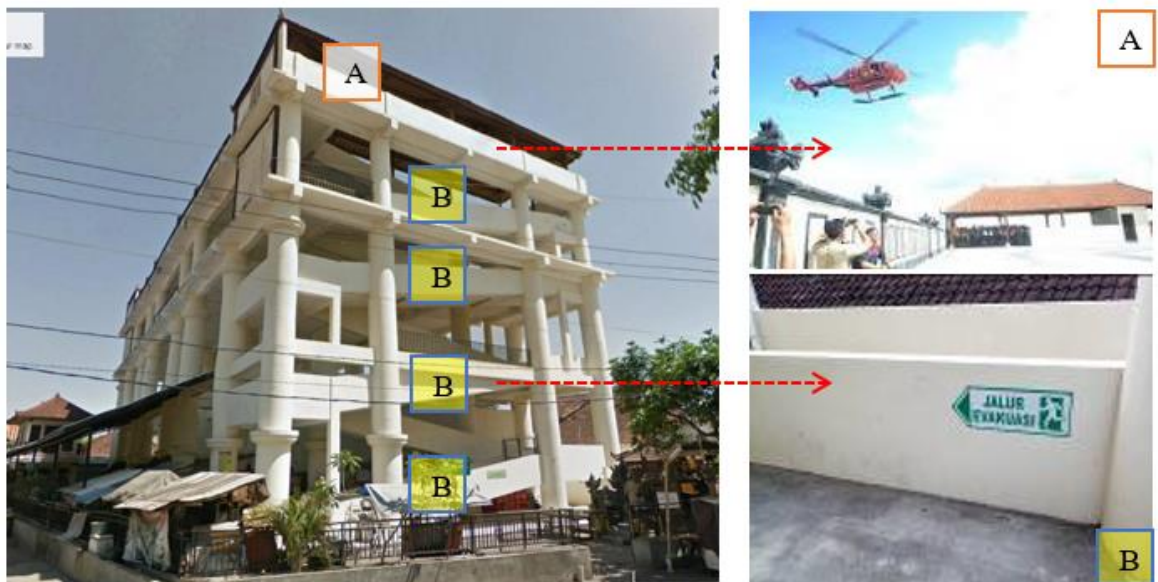
Figure 12: Placement of Ramps and Heliport in TES Tsunami Building, 2020 Source: Researcher Documentation
