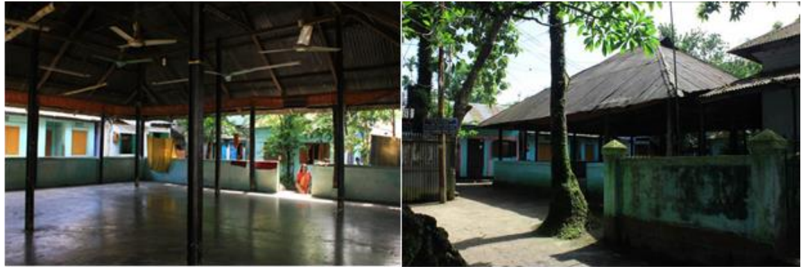
Figure 5 Interior & exterior spaces of Shamsundar Akhada, Lamabazar, Sylhet.
