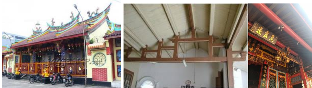
Figure 2: Roof shape, ornament, and color ( source: https://www.academia.edu cited May 2019 & survey result May 2019)
