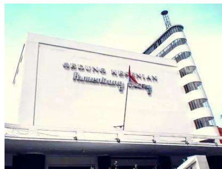
Figure 1. Rumenteng Siang arts building
